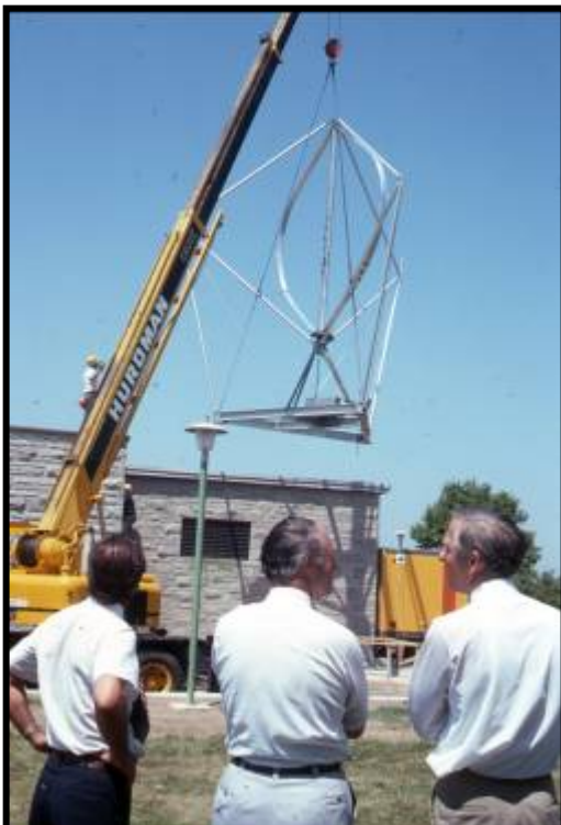
Figure 6 - Installing the turbine at the Rideau Falls model home. The turbine is now in the collection at the Canada Science and Technology Museum in Ottawa, Ontario. (1984.1223)
