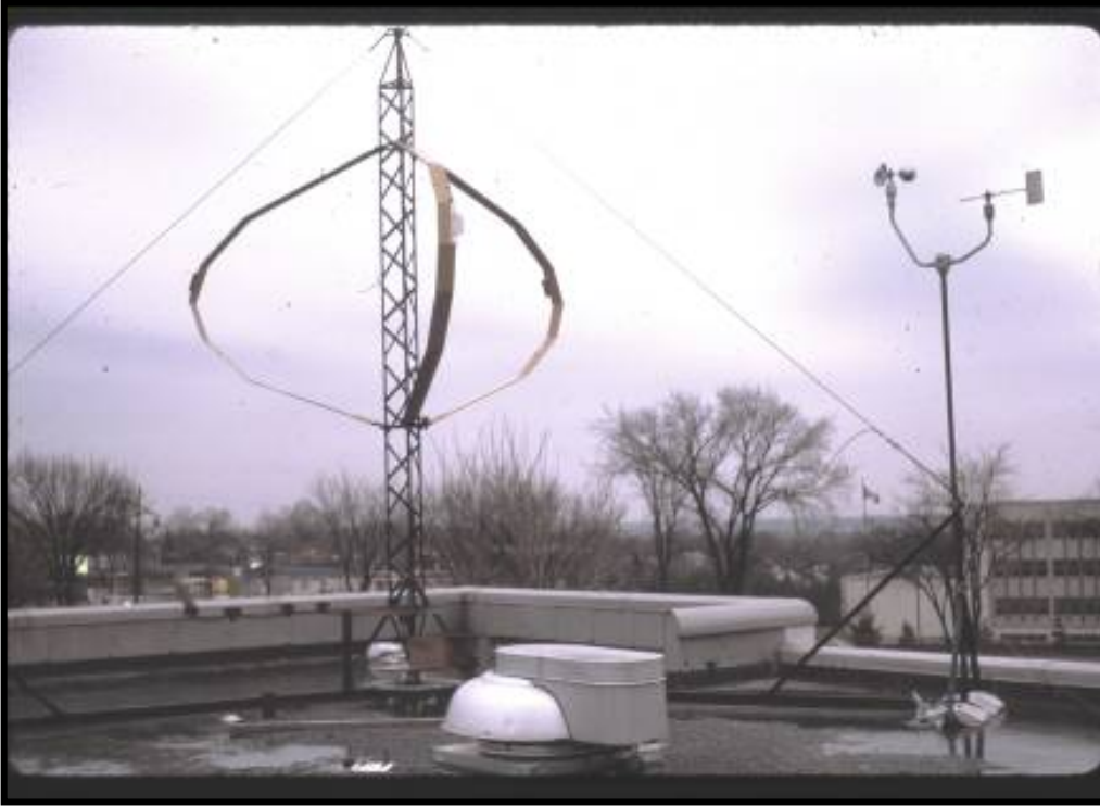
Figure 3 - The first Darrieus type vertical axis wind turbines developed by Raj Rangi and Peter South. This turbine was erected on the top of one of the research buildings as the National Research Council of Canada.
